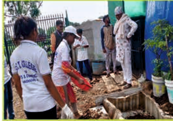
Kitchen Garden at Shelter Home "Growing hope through sustainable initiatives."
