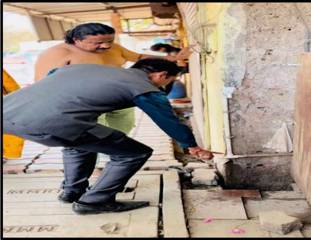
Leakage repaired with M Seal
