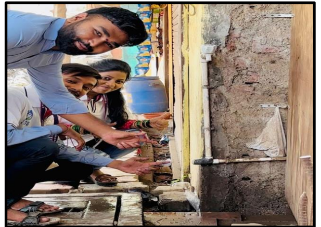
Water leakages observed by students of SST College
