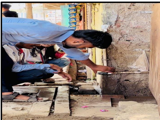
Leakage repaired with M Seal
